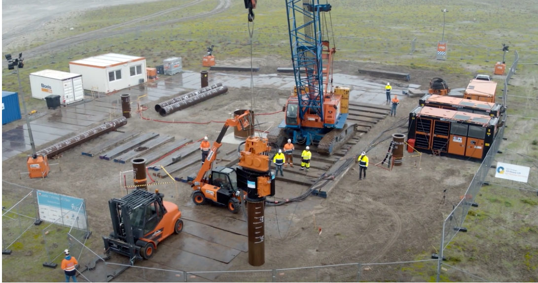
Figure 2: Installation test of a pile driven by the GDP method.
